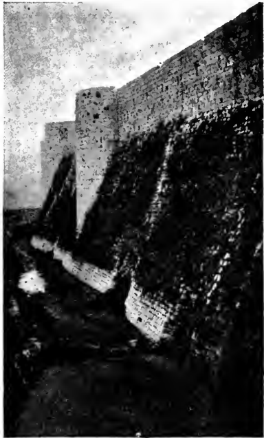
ḲAL'AT EL HUṢN, WALLS OF THE INNER ENCEINTE
